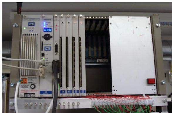
Fig 2: The new CTI system (In order from left: Power Supply, CPU, Interface card, 4 Analog 8 Channels IN/OUT cards)
